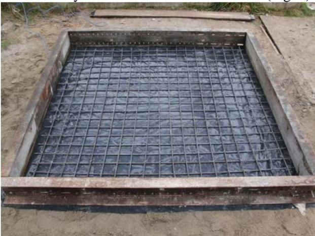
Fig. 2 Reinforcement of the slab
