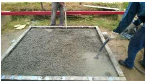
Fig. 2: Concreting of tested foundation slab
