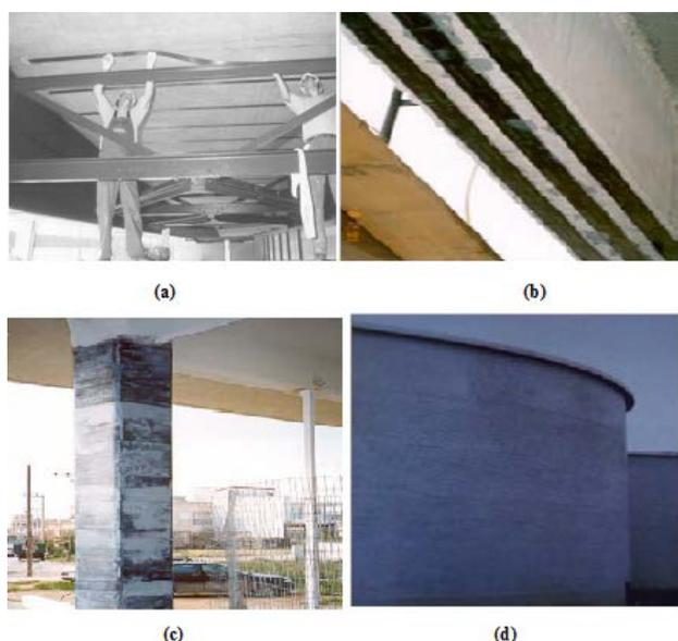
**Fig.1** Typical FRP applications as strengthening materials of RC structures: (a) flexural strengthening of slab; (b) flexural strengthening of beam; (c) shear strengthening and confinement of column; (d) wrapping of concrete tank.
