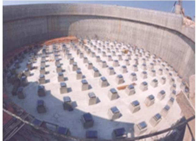
Fig.10: Overview of Seismic Isolators of NPP Structure, [17].
