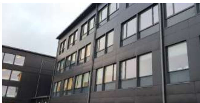
Picture 3 Continous measurement at facade of office building
