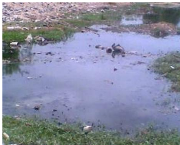
Fig. 1. Unlined Wastewater Channel, Soje
