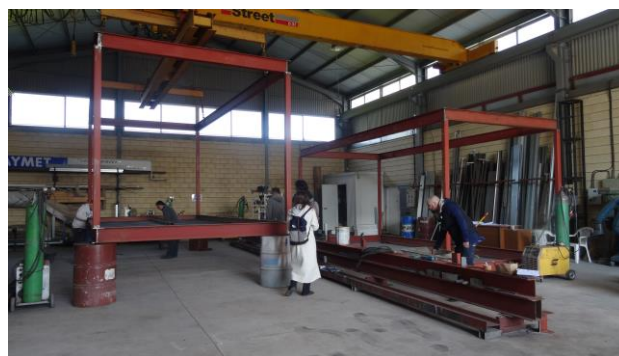
Figure 4 Images of the assemblance process of the structural frame of the units, which is consisted by two main units, thus forming a small family house.
