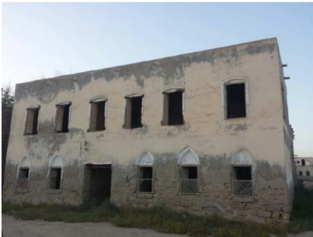
Fig.2 Dwelling exterior view – street façade
