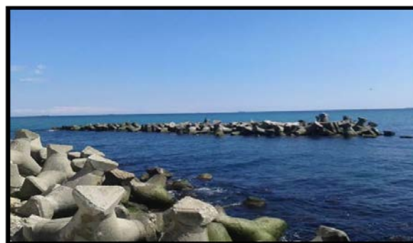
Figure 1 – Detached Breackwaters – Longitudinal structures
