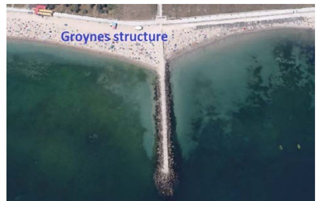
Figure 11 – Mamaia Bay, groyne structure [Google Earth]
