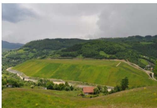
Fig.3. Achievement of closure and greening layers of Gura Rosiei TMF
