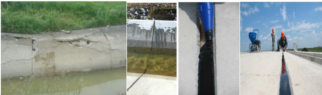
Pictures 4, 5,6&7. Current status of a partially restored canal and the rehabilitation canal with the Fuga materials
