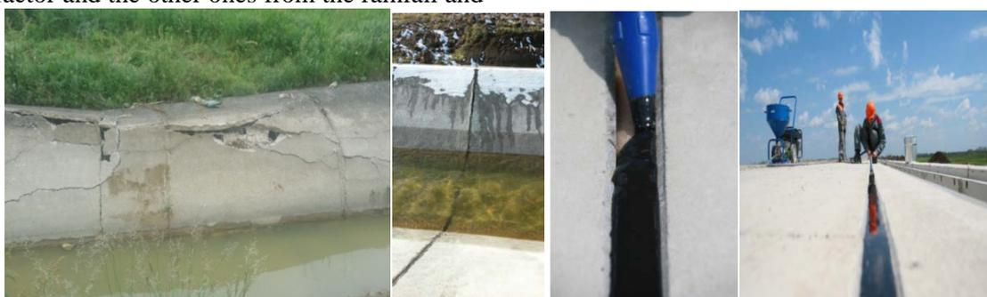
Pictures 4, 5,6&7. Current status of a partially restored canal and the rehabilitacion canal with the Fuga materials
