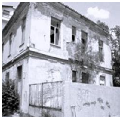
Fig. 5: Office building view [5]
