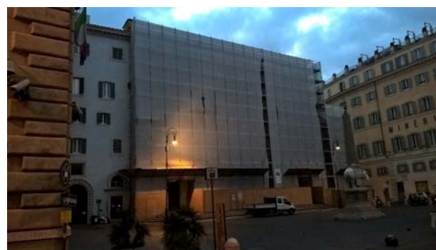
Fig. n.2 Scaffolding on the facade of S. Maria sopra Minerva, photo: S.Coccoli
