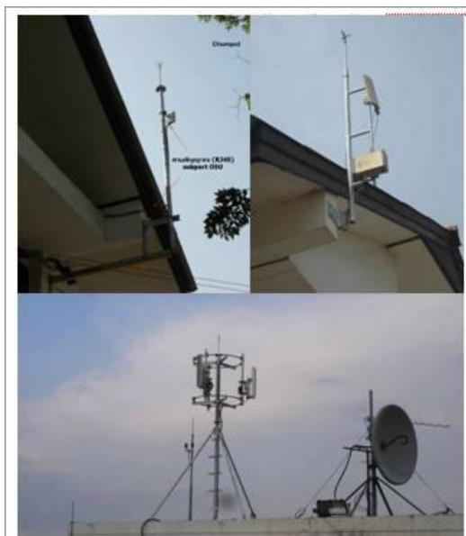
Figure 17. The 3-sectors Wi-MAX's antenna at Health center and MSMC building.
