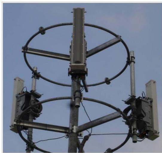
Figure 18. The 3-sectors BTS antenna installation.
