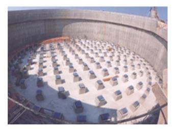
Fig.10: Overview of Seismic Isolators of NPP Structure, [17].
