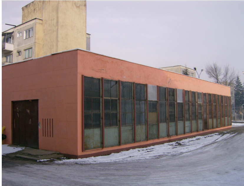
Fig.9 Thermal station ASTRA Brasov before installing the solar panels.
