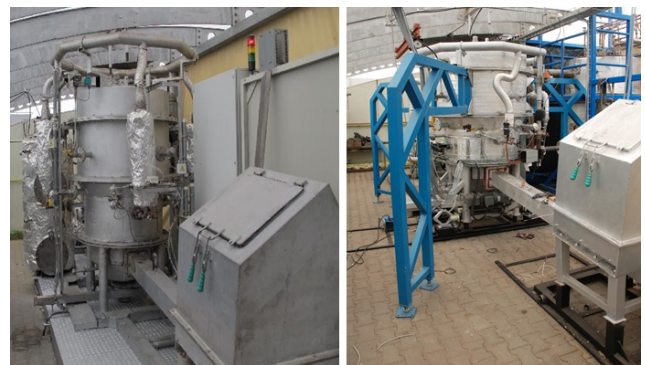
Fig. 5. Generator before and after reconstruction
