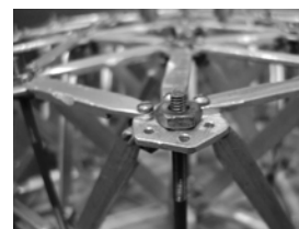
Fig. 2. Screws and washers in the frame of a solar concentrator
