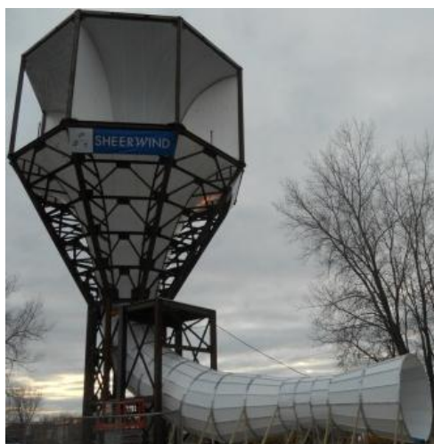
Figure 5. Invelox demo tower [13].
