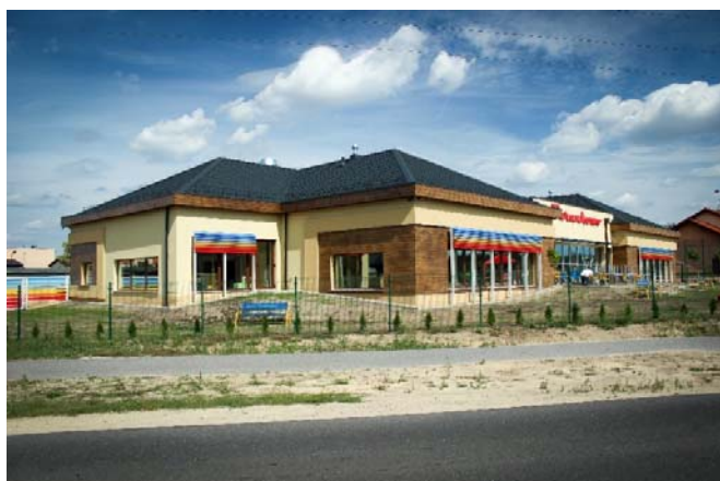
Fig. 12 Tested kindergarten and nursery in Baranów [3]
