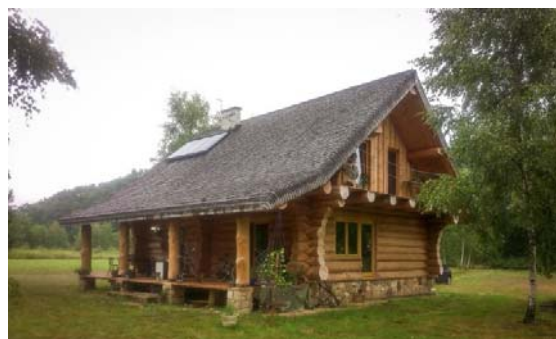
Fig. 14 Tested house built of wooden logs [3]
