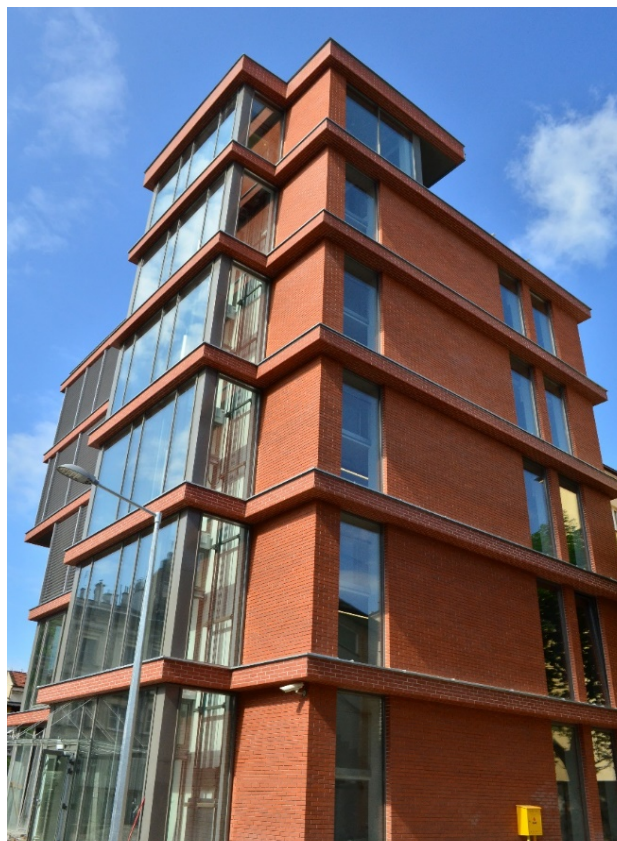
Fig. 5 View of the MLBE building. Laboratory of energy efficient technology
