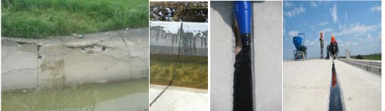
Pictures 4, 5,6&7. Current status of a partially restored canal and the rehabilitation canal with the Fuga materials
