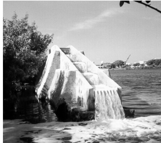
Fig. 3. Structure built in the lagoon aeration Bojórquez, Cancun, Mexico.
