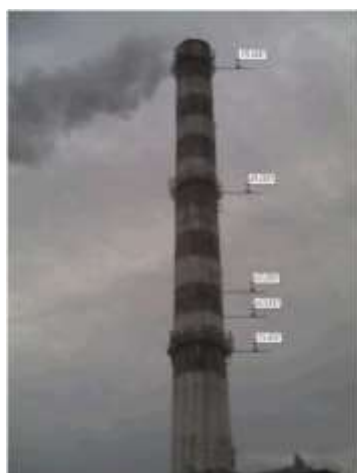
Fig. 8. General view of the industrial chimney 120 for PTVM-100 boiler units
