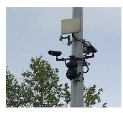
Fig.1 NIR cameras on traffic intersections
